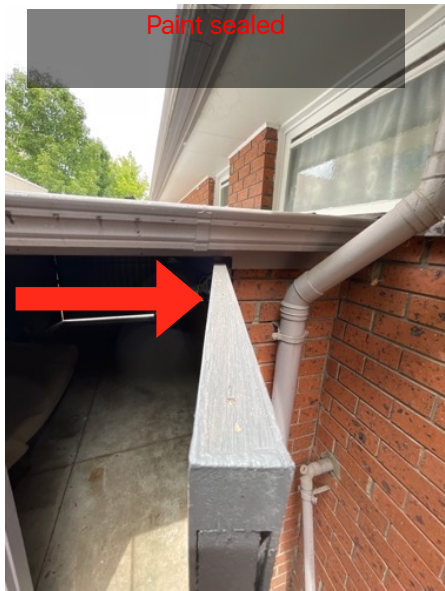
Moisture ingress damage
